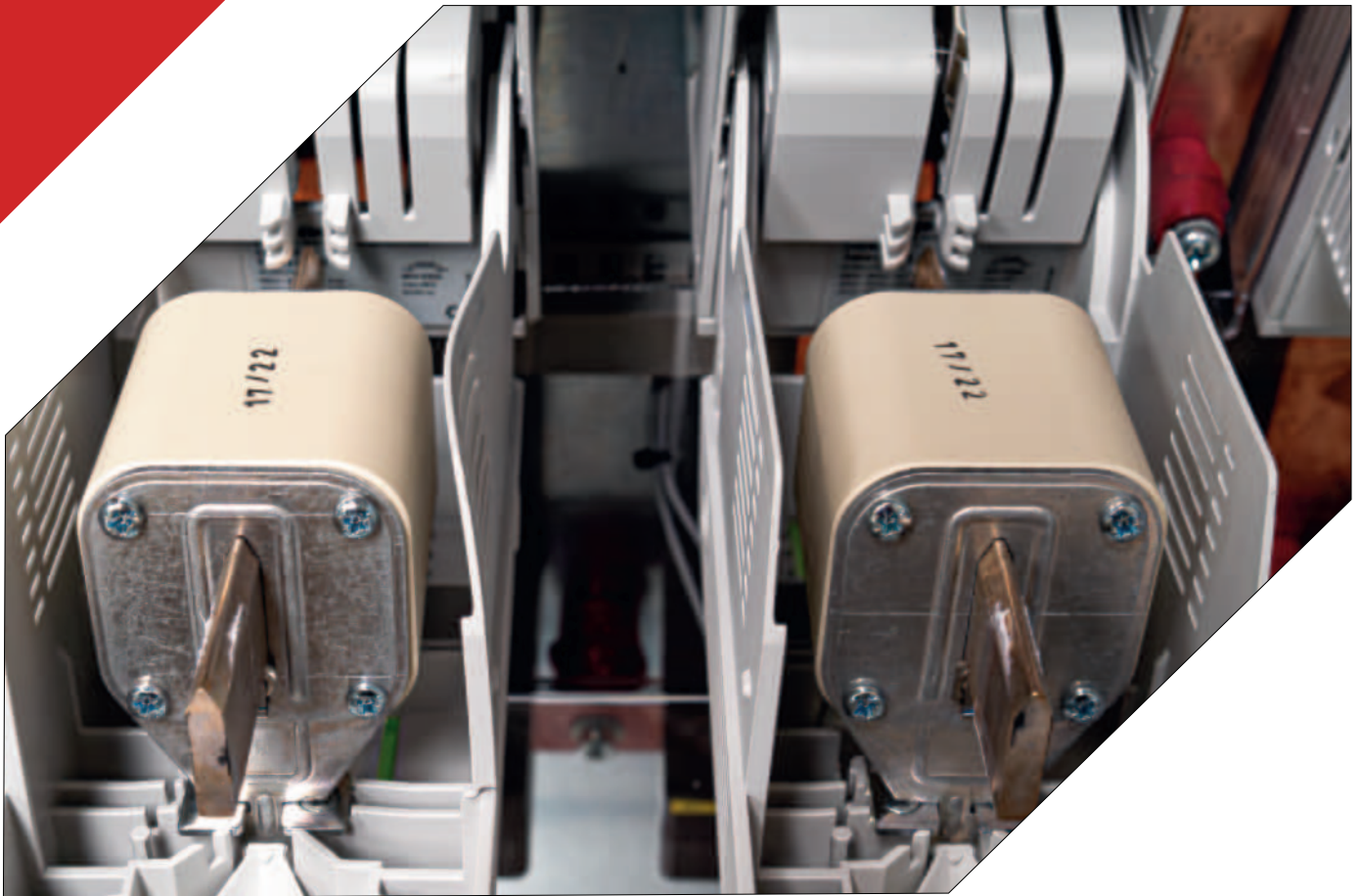
Output fuse open, one for each electrode
